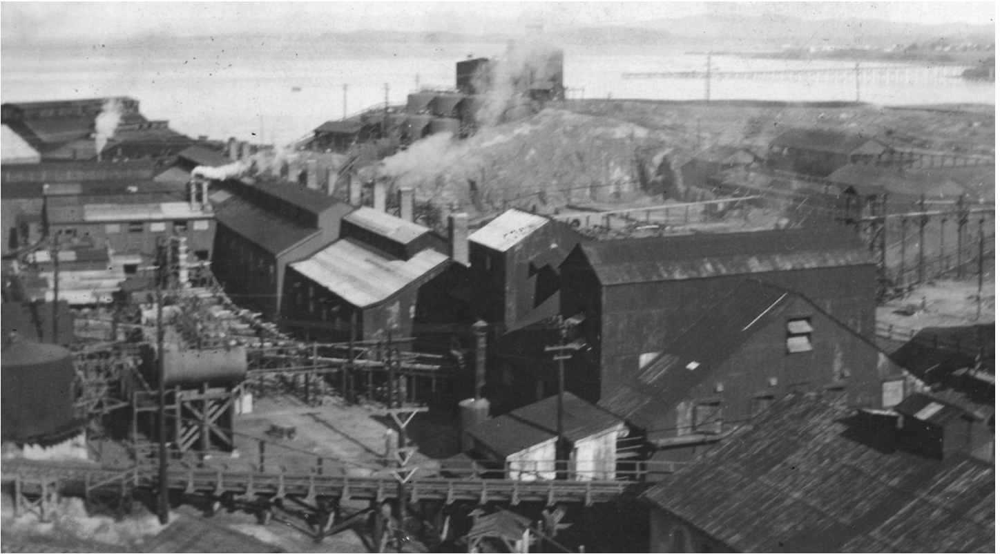
Hercules Powder Works acid area and wharf. (Photo courtesy Steve Lawton).
