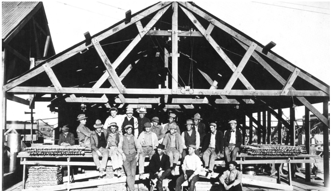
Workers at the Hercules Powder Works Pipe Shop.
