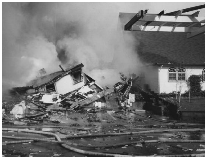
Remains of the Second Fiddle thrift store, with the Pythian Castle building at the right, after the February 17, 1998, explosion. Photo courtesy of Adila Araya.
