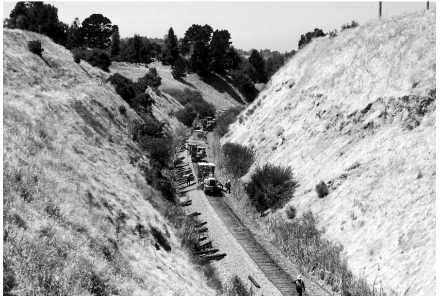
Westward view of the daylighted portion of the tunnel leading into Pinole. Santa Fe's noted Navajo Track Crew is working the area in on August 8, 1996. Photo by Jack Meehan.
