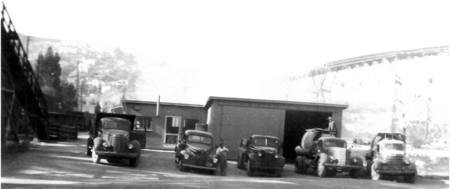
Sugar City Building Materials in the company's Crockett yard in 1933.
