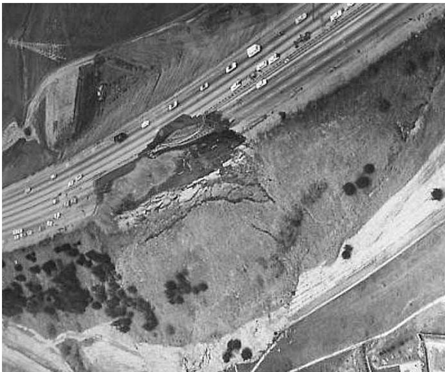
I-80 collapse in Pinole, May 12, 1969.
