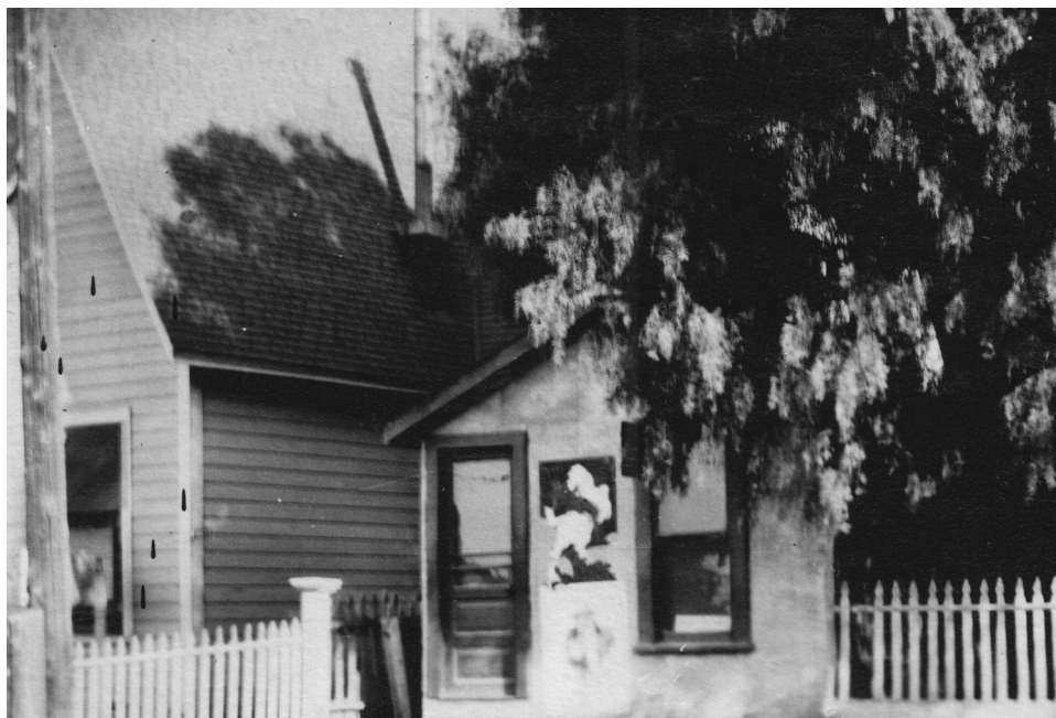
Pinole's first tin-roof library building.
