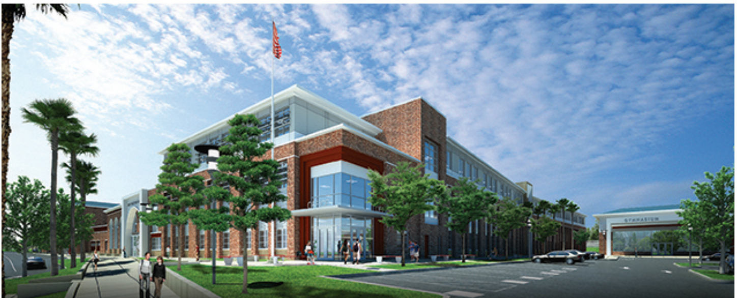
View of the new Pinole Valley High School Administration building and gymnasium.
